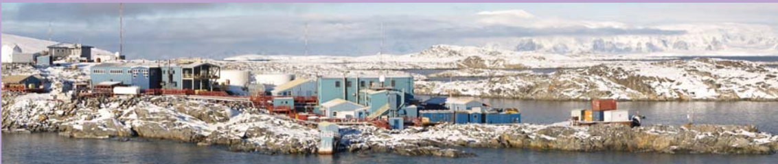
Palmer Station, located midway down the Antarctic Peninsula on Anvers Island, is the smallest of the three stations operated by the U.S. Antarctic Program. Credit: Patrick Rowe, National Science Foundation
